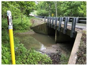
The Pauling-Goodenow Road underpass at CSX/UP railroad is in the floodplain north of the road. Although the underpass has not had a reported closure due to flooding, maintenance personnel often need to clean gravel out of the grates following a storm.
