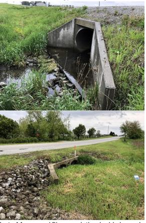
Crete-Monee Road: At Crete-Monee and Pinewood, the double box culvert has undesirable skewed geometry, was observed to have a highwater level (i.e. freeboard issue), has many nearby utility poles, and has a nearby CMP culvert beneath Pinewood.
