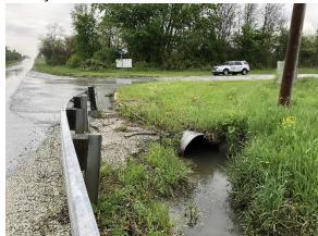
Pauling Goodenow Road: The Pauling-Goodenow double box culvert at the Rock Creek is in IDOT's Structure Summary Reports. There are narrow shoulders, pipeline on the south side, and utility poles on the north side. The east box is silted up, suggesting a drainage issue.
